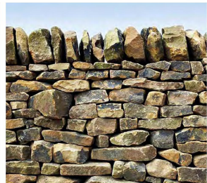
Reinstated & New Drystone Walls using Site-Won Stone
