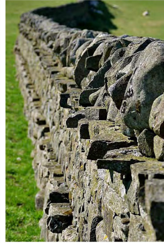
Traditional Drystone Wall with Throughstones
