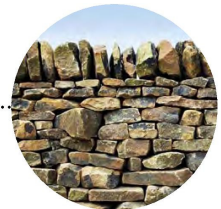
Drystone Wall using Site-Won Stone
